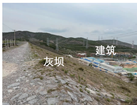
图 11 灰坝坝脚附近房屋建设 Fig.11 Construction of houses near the foot of an ash dam
