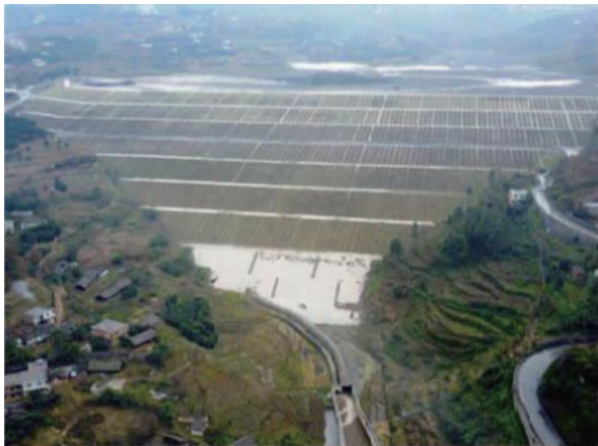
图 14 贮灰场脱硫石膏与粉煤灰混合料筑坝 [11] Fig.14 Damming with desulfurized gypsum and coal ash mixture in coal ash storage facility [11]
