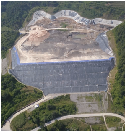
图 15 后龙山贮灰场纯石膏筑坝 Fig.15 Damming with pure gypsum in Houlongshan coal ash storage facility
